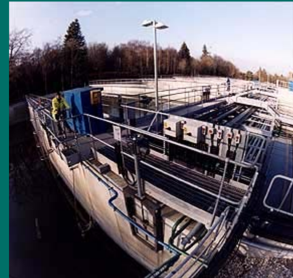
The North Ponds Water Management System.
