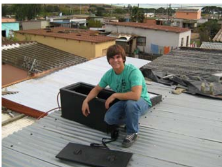
Jaco duToit installing a prototype low cost solar water heating unit
