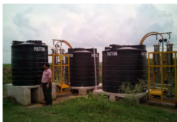
Figure 1. The Arsenic Removal Plant presently used by the CGCRI used in rural areas in West Bengal. The ATP combines adsorption on iron oxide and ultrafiltration using a ceramic filter.
