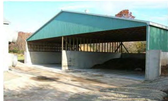
Poultry manure storage facility
