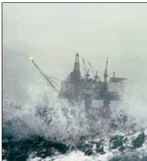
ABOVE: "GULLFAKS C" BATTERED BY STORM-FORCE SEA (Photo credit: Arnulf Husmo-Stone, Getty Images)
