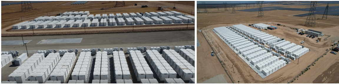
Figure S27: The AES Luna Battery (100 MW/400 MWh) and Lancaster Area Battery (127 MW/508 MWh) with a combined rating of 227 MW/908 MWh are not visible on satellite images yet but locations are included here for future comparisons. Construction can be seen on wego.here.com satellite images. Location: 34°41'5.04"N 118°18'17.91"W
