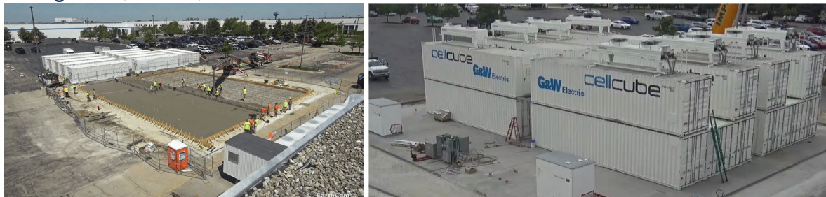
Figure S65: Satellite images of the 2 MW/8.5 MWh site are not up to date, according to the company, the site uses four FB500-2000 units with a footprint of 450 m 2 , corresponding to around 19 kWh m -2 . Location: 41°40'24.86"N 88° 4'13.68"W
