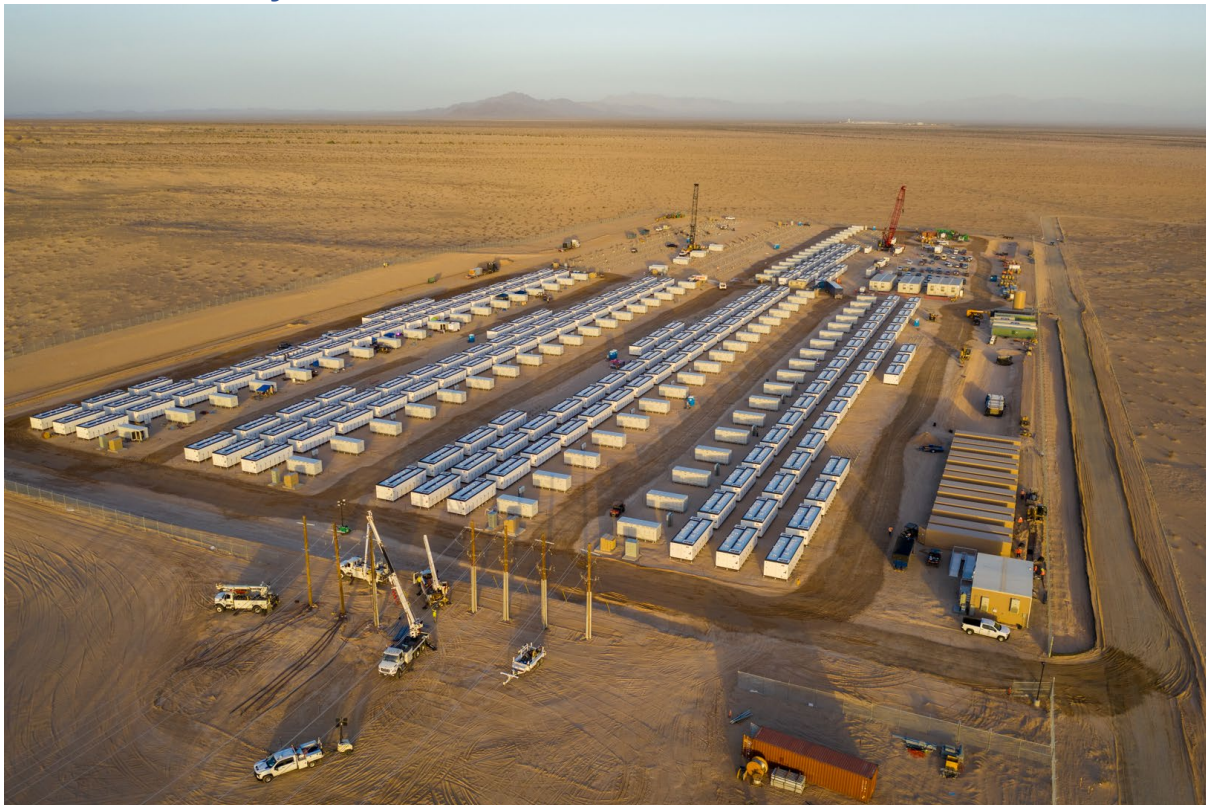
Figure S28: The Crimson Energy Storage Project is the largest BESS to reach operation in a single phase so far, rated at 350 MW/1400 MWh. It is not visible on Google Earth yet but is included here for future comparisons. Location: 33°34'13.27"N 114°49'47.15"W
