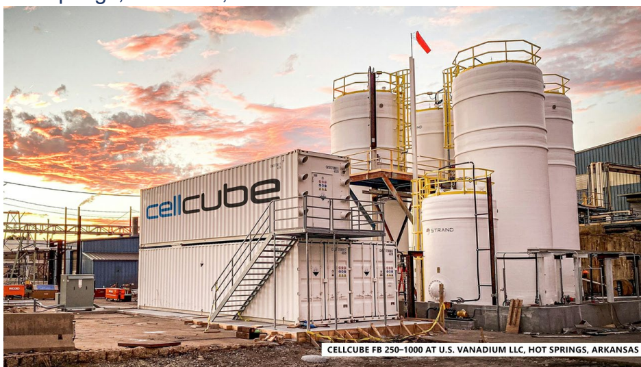
Figure S66: Satellite images of the 0.25 MW/1 MWh site are not up to date, according to the company, the site uses a FB250-1000 unit with a footprint of 60 m 2 , corresponding to roughly 17 kWh m -2 . Location: 34°28'1.45"N 92°56'52.39"W
