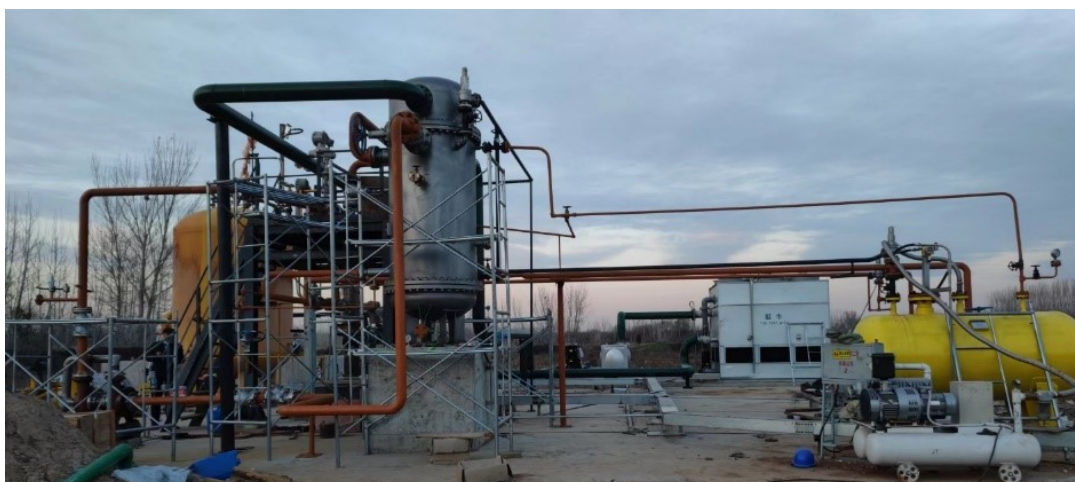
Extended Data Fig. 1 Photo image of the SLGHP geothermal system built in Xiong'an New Area, China. This pilot SLGHP geothermal system underwent two sets of tests for heat extraction and power generation, respectively.
