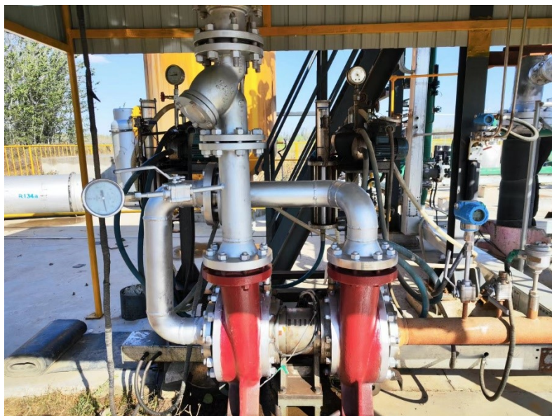
Extended Data Fig. 5 Photo image of the SLGHP direct-driven power generation system. The ammonia vapor produced by the heat pipe directly enters the first stage turbine, and then goes to the second stage. After driving the turbine, the ammonia exhausting the turbine enters the condenser through the orange pipeline on the right-hand side of the photo.
