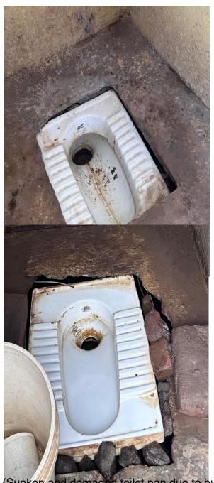
(Sunken and damaged toilet pan due to burrowers needs to be replaced)
